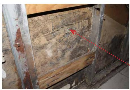
Very quickly, the mold was revealed to be substantial throughout the area originally identified as suspect. It is common to see vast colonies of mold growth behind drywall that frontally appears minimal or mold free.
