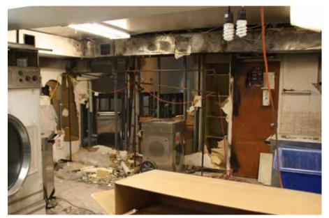
The site sustained serious fire and smoke damage and was in a state of disaster, with structural materials charred, sooty or displaced entirely. The disengagement of the materials is what revealed the presence of mold, as well as an obvious repeated contact with water in the past.
