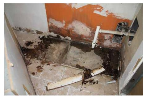
In this area where a sink was removed, it is definitely in need of cleaning. However, when the material was inspected closely, it became clear that mold had taken hold here.
