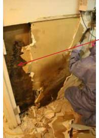
Proper procedure indicates the cutting of wall material a minimum of two feet above the common height of the mold growth, then the complete removal of the board below.
